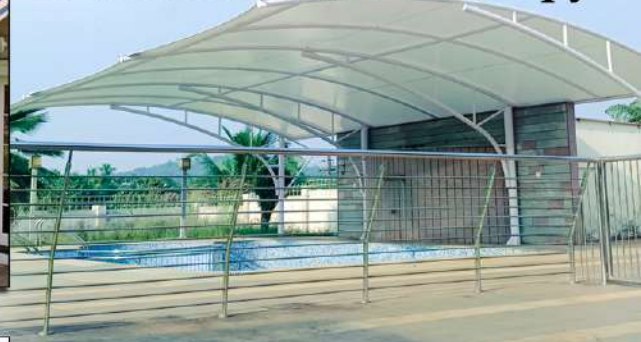
Tensile Structured Canopy
